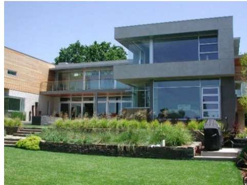
Twenty-First Century Contemporary: Orthogonal volumes with different wall textures or materials creating a sculptural effect.
