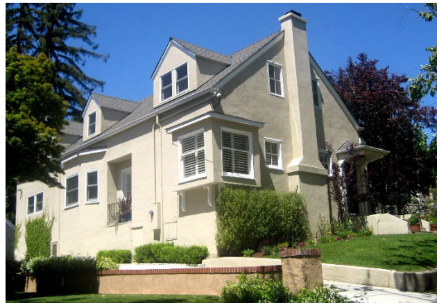
The new second floor addition uses the mix of window styles found at the existing first floor.
