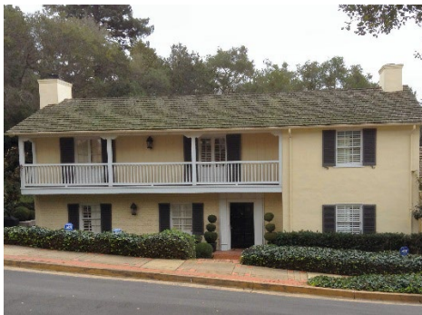
Monterey Colonial: Shallow roofs, exposed wood rafters, second floor veranda with railings.
