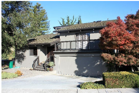
Split Level: Tri-level with intersecting roofs with asymmetrical windows and entry.
