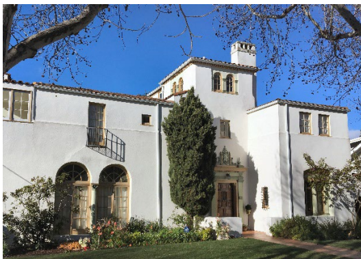
Spanish Revival: Low pitched tiled roof, little or no overhang, deeply recessed windows and doors.
