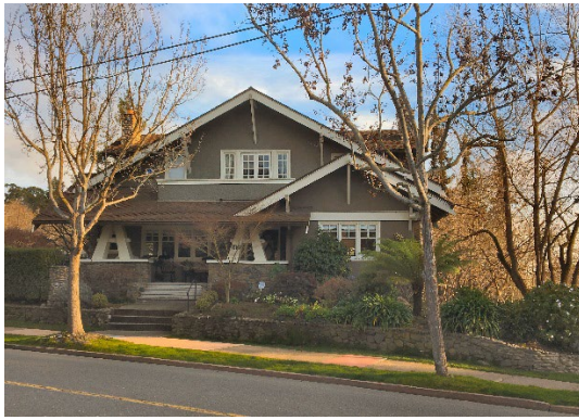
Craftsman: Low pitched gable roof with deep overhangs and exposed roof rafters.
