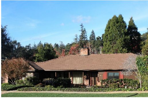
Styled Ranch-Colonial Revival: Prominent hip or gable roof, revival styled walls, windows and details.
