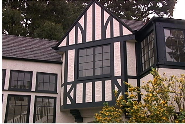
Windows at the addition to the left are consistent with the existing windows to the right.
